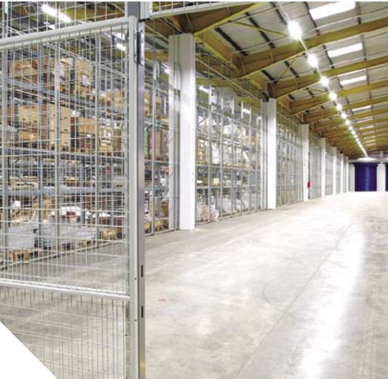
FlexiStore is used here to divide a section of the IKEA Leeds store in England.
