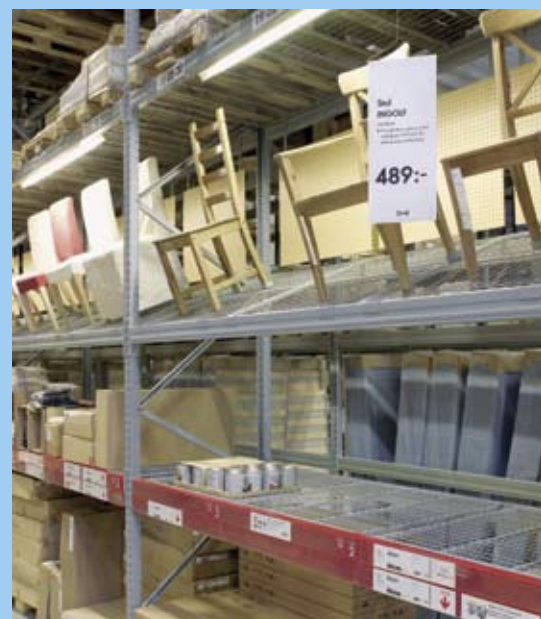
► ShelfStore in pallet racks at the self-service store at IKEA in Jönköping, Sweden.
