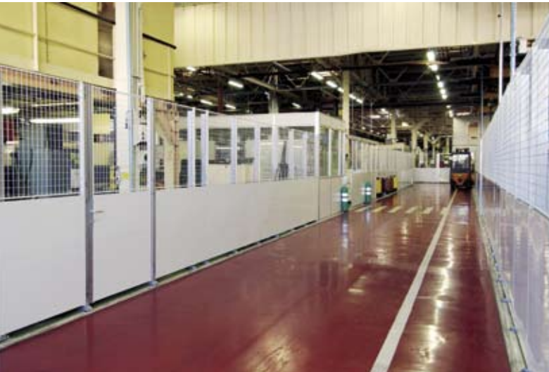
FlexiStore in sheet metal and mesh enclosing a new operation & maintenance department at Renault Cléon in France.
