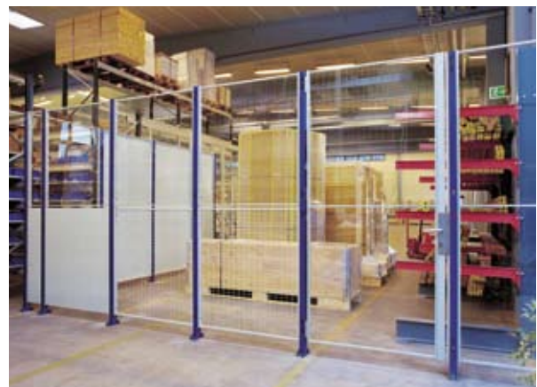
FlexiStore plastic and sheet metal dividing a warehouse. A hinge door with cylinder lock is used.
